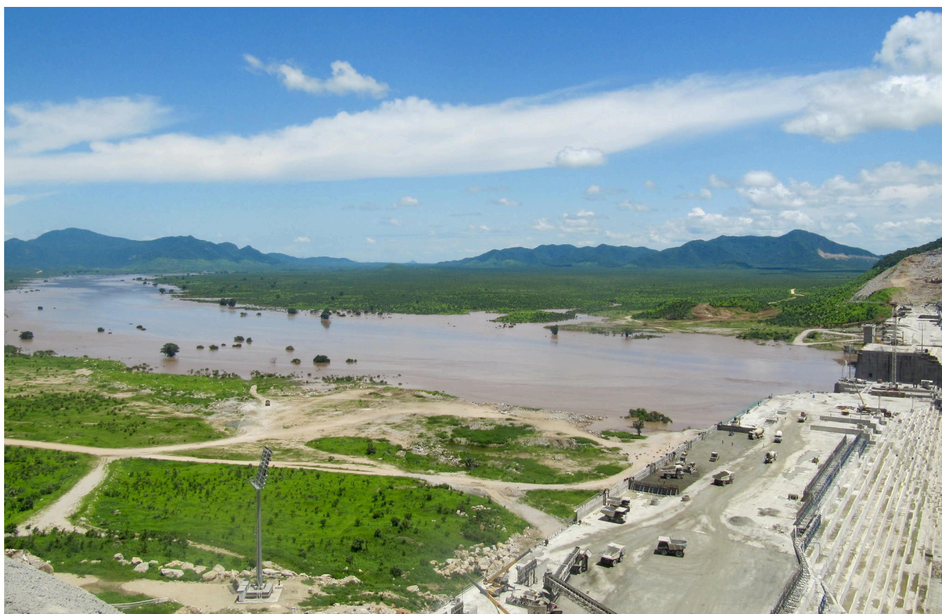
Construction of the Grand Ethiopian Renaissance Dam. Credit: CC/Ana E. Cascão
